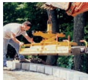
Laying Clamp for retaining wall units RWC
